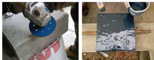
Fig 7. View of Grinder Applying Epoxy on Concrete
