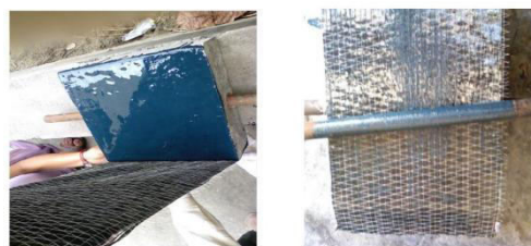
Fig 8. Placing Carbon Fiber Sheets Rod Used for Smoothing
